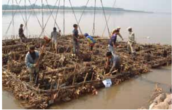
Pic. 5 SODA mattress fixing using crane machine
