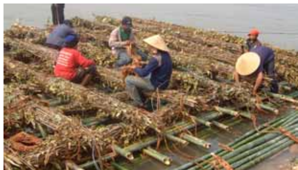
Pic. 6 SODA mattress assembling on water
