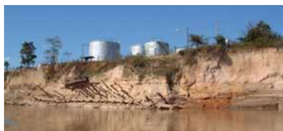
Pic 1 Eroded riverbank in front of oil tank in Vientiane City
