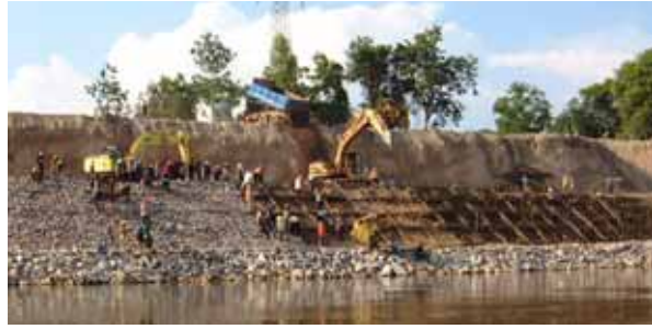
Pic. 4 Pilot works at Dongphosi site on Mekong river
